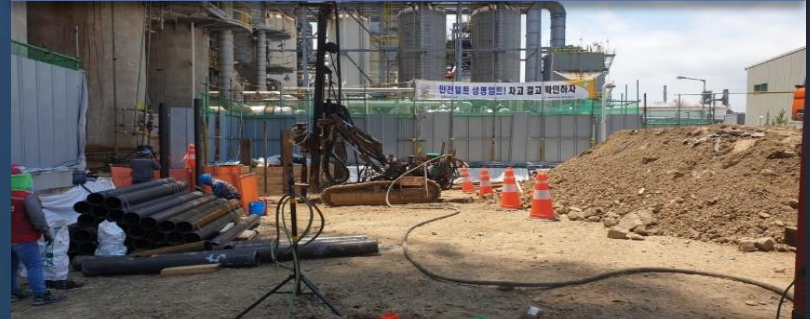
울산S-OIL #2 ARO H2 RICH GAS COMPRESSOR INSTALLATION
